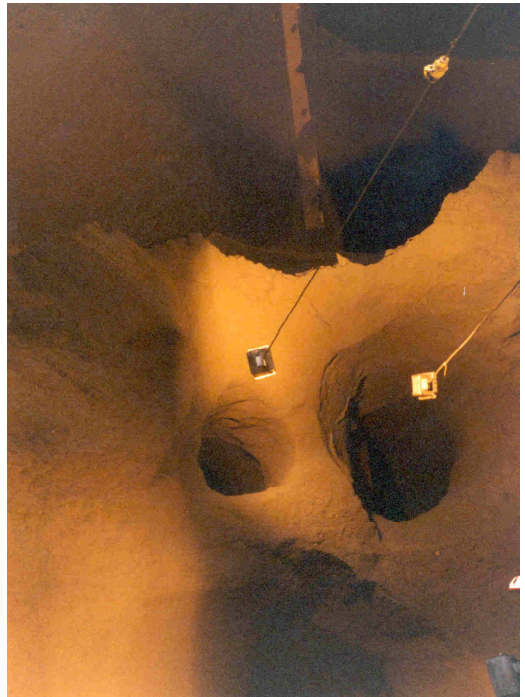
Rat holes in the bunker BEFORE fitting Ajax inserts
